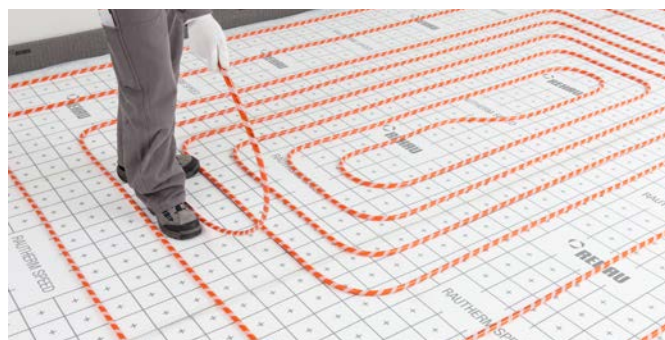
Abb. 4-17 Klettsystem RAUTHERM SPEED
